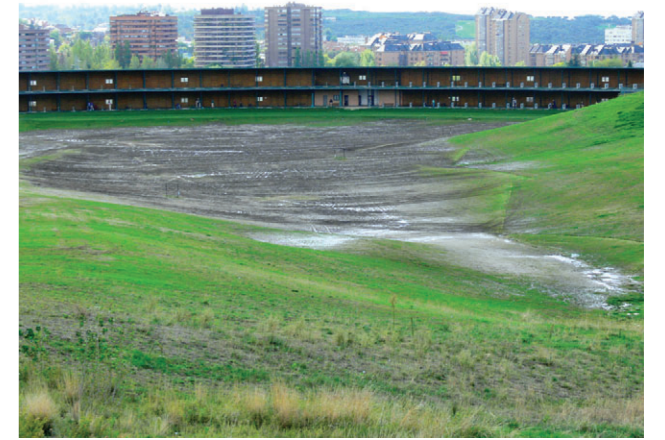
Poor drainage reduces potential revenue
