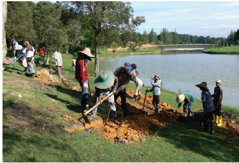
Digging drains, Malaysia
